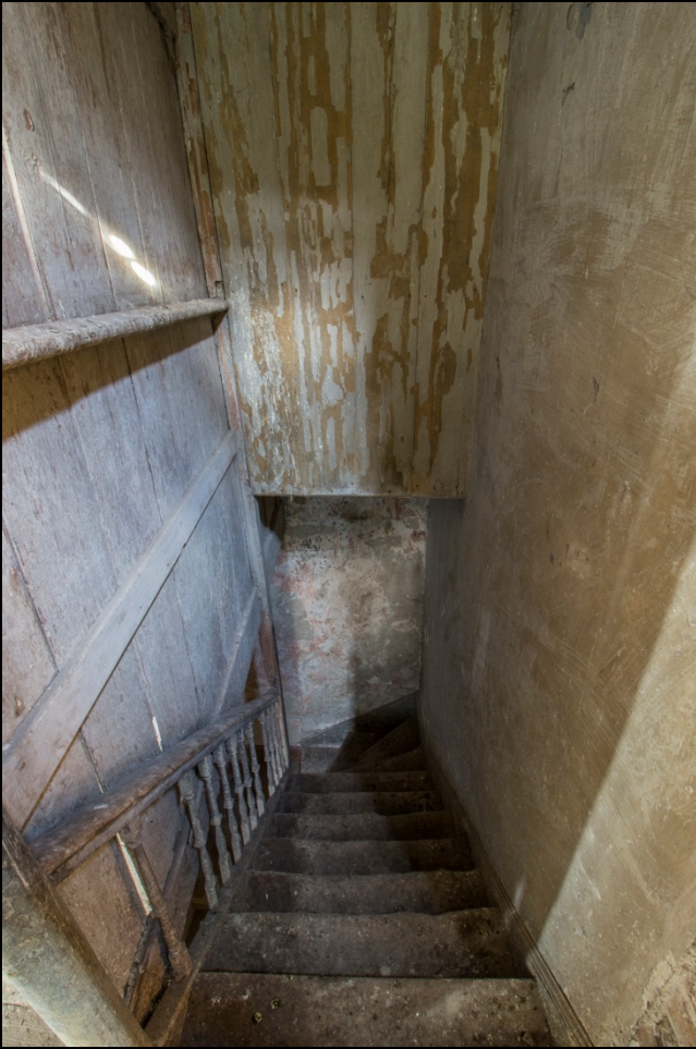
Looking down the stairs from first floor
