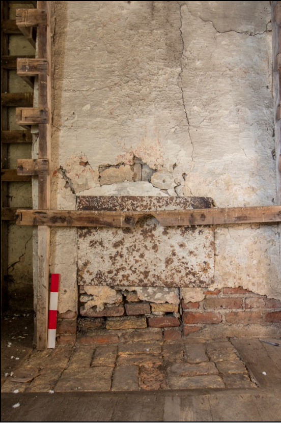
Bricked up chimney in 2 nd floor room
