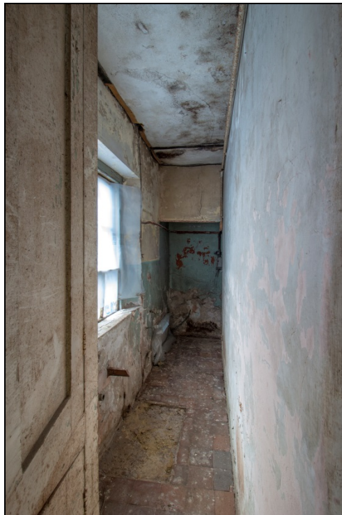
Ground floor area with modern "chiller room"
